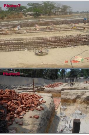
COP-180: 44 nos. cast in situ piles out of 75 nos. have been cast so far. Each pile has a length of 20.1 m and diameter of 500 mm. Preparations for casting of situ piles is in progress (Photo:9).
