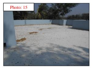
Patent Stone Casting: Completed at ground floor of NOAE-313 & NOAE-314. The ground floor of NOAE-313 has undulated rough surface instead of levelled smooth surface (Photo: 16). Curative measures should be taken.
