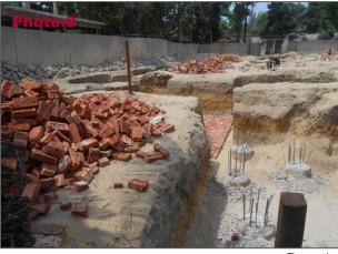
COP-180: 44 nos. cast in situ piles out of 75 nos. have been cast so far. Each pile has a length of 20.1 m and diameter of 500 mm. Preparations for casting of situ piles is in progress (Photo:9).
